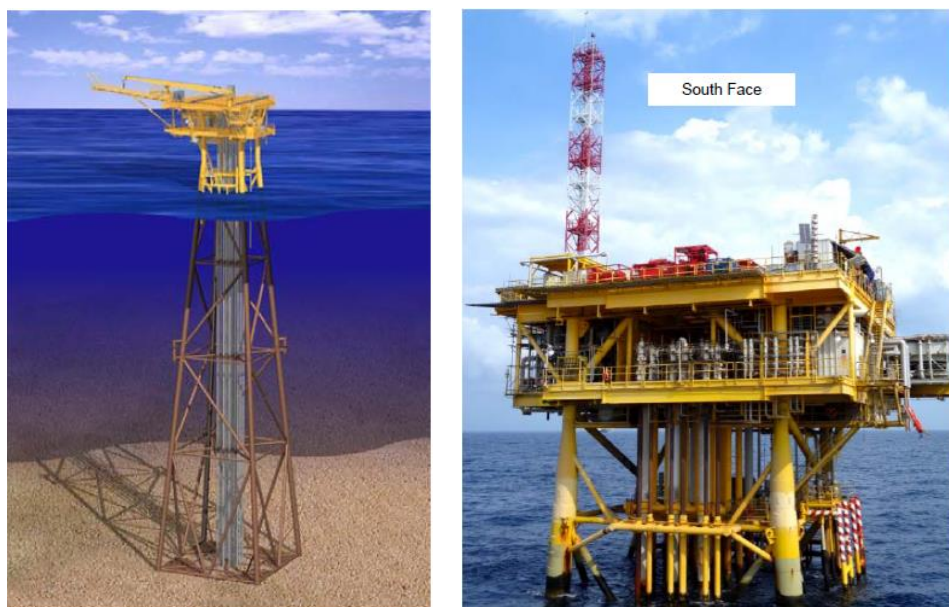
Figure 5 Typical wellhead platform in the Gulf of Thailand [Ref. 2]
