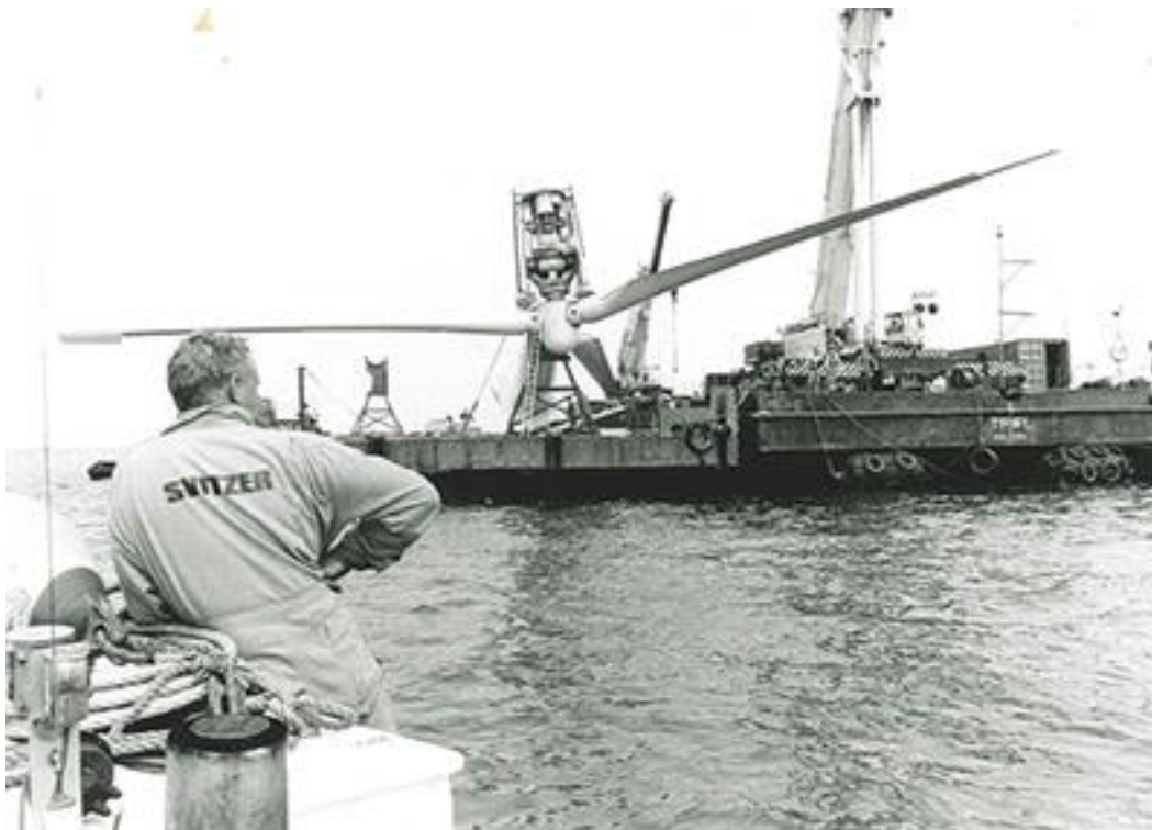
Figure 3. Installation work being carried out on the first wind farm at Vindeby (source: Windeurope [1])
