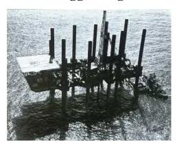
The Offshore Rig 51 is generally accepted as the first mobile offshore drilling jack-up and was delivered in 1954. It had 10 legs, each of 6 feet in diameter, and used the Delong type pneumatic jacking system.
