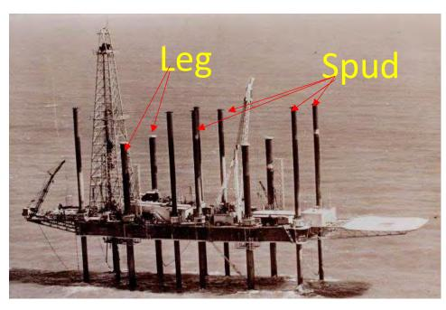
12 legs. But that would be (marginally) misleading. The unit was originally built as two barges, each equipped with four spuds and two legs. The hull of the platform wasn't buoyant, so it was towed to location on the buoyancy of the lower barge, or mat. Once on location, the four spuds were
