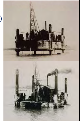
Port Weller Harbour Drilling Jack-Up used winches to raise the hull (1914)
