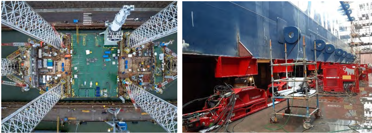
Figure 10: Alignment prior to skidding (left), skidding of midsection (right)
