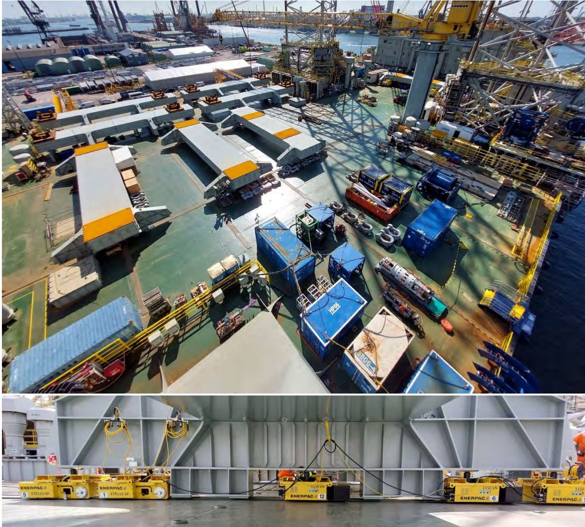
Figure 5: Deck transfer system grillages and tracks (top), Trolleys under the grillage (bottom)
