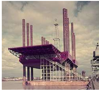
(a) Old oil and gas jack-up with tubular legs
