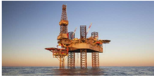
(b) Modern oil and gas jack-up with truss legs
